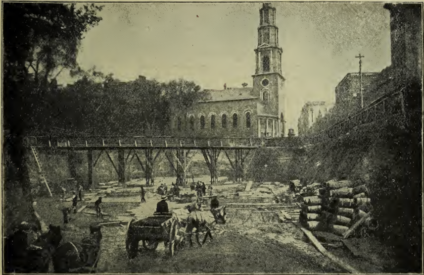
WORK ON SECTION THREE, LOOKING NORTHERLY, MAY 14, 1896.
